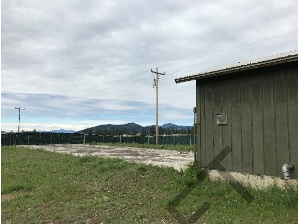
Reservoir with Pump House
