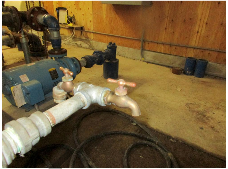
Photograph 12: Smooth nosed sample tap
