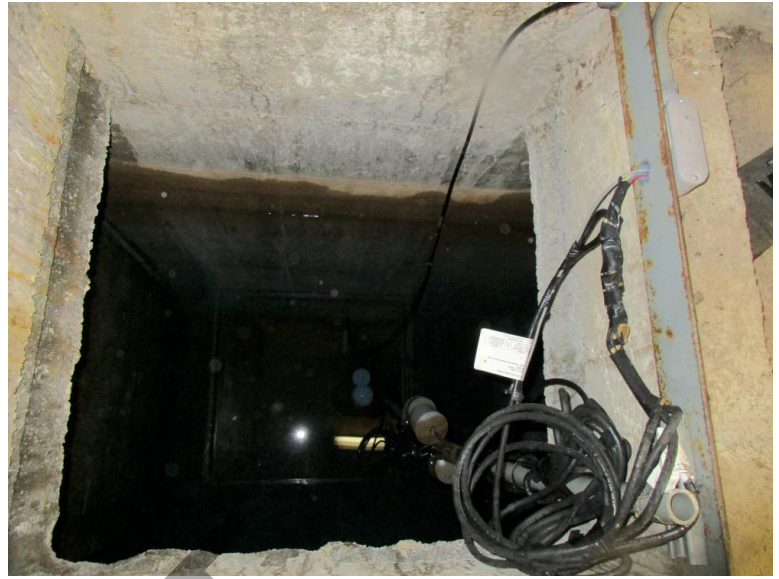
Photograph 16: Inside view of hatch into storage tank
