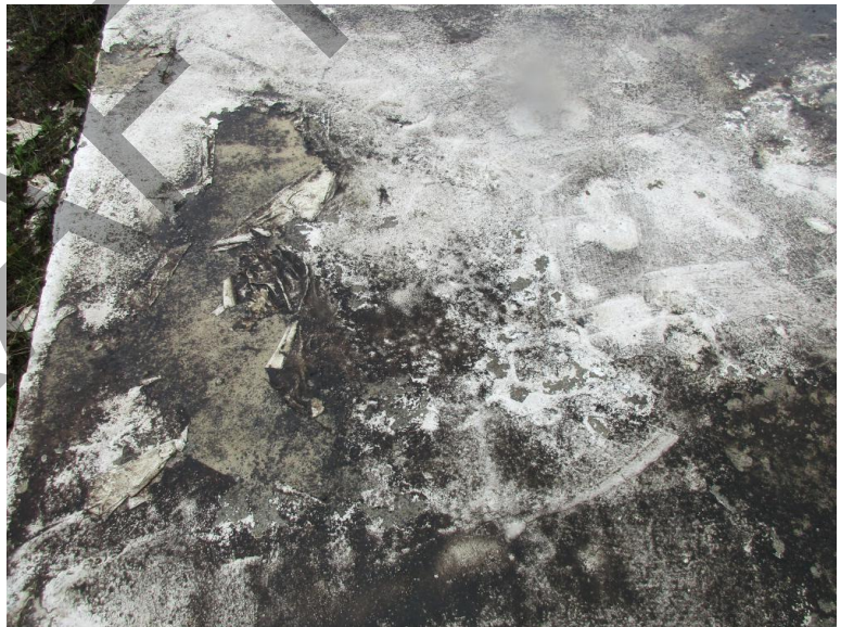
Photograph 4: Storage tank roof
