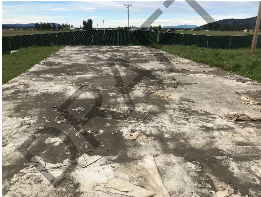
Top of Reservoir
