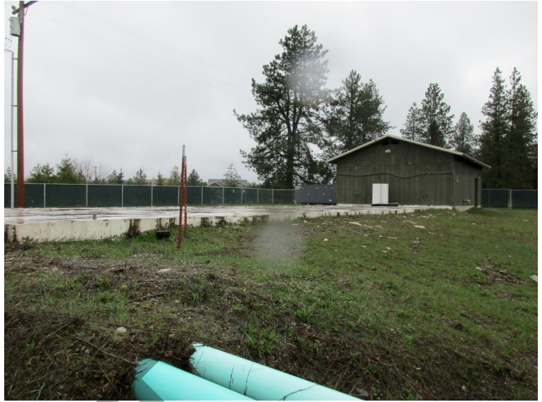
Photograph 24: View of pump house and top of storage tank
