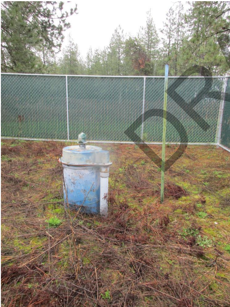
Photograph 25: Well 1 located across street from pump house
