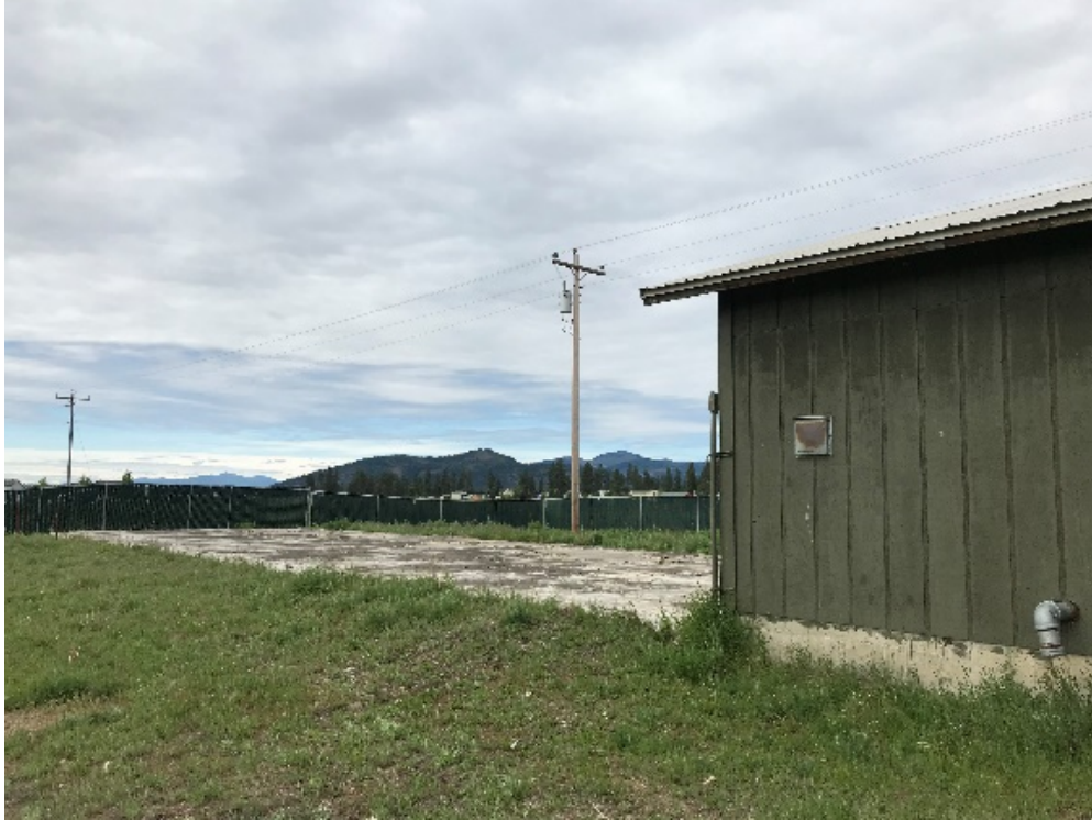
Reservoir with Pump House
