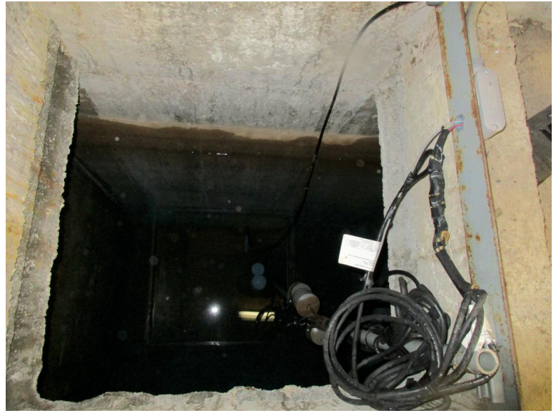
Photograph 16: Inside view of hatch into storage tank
