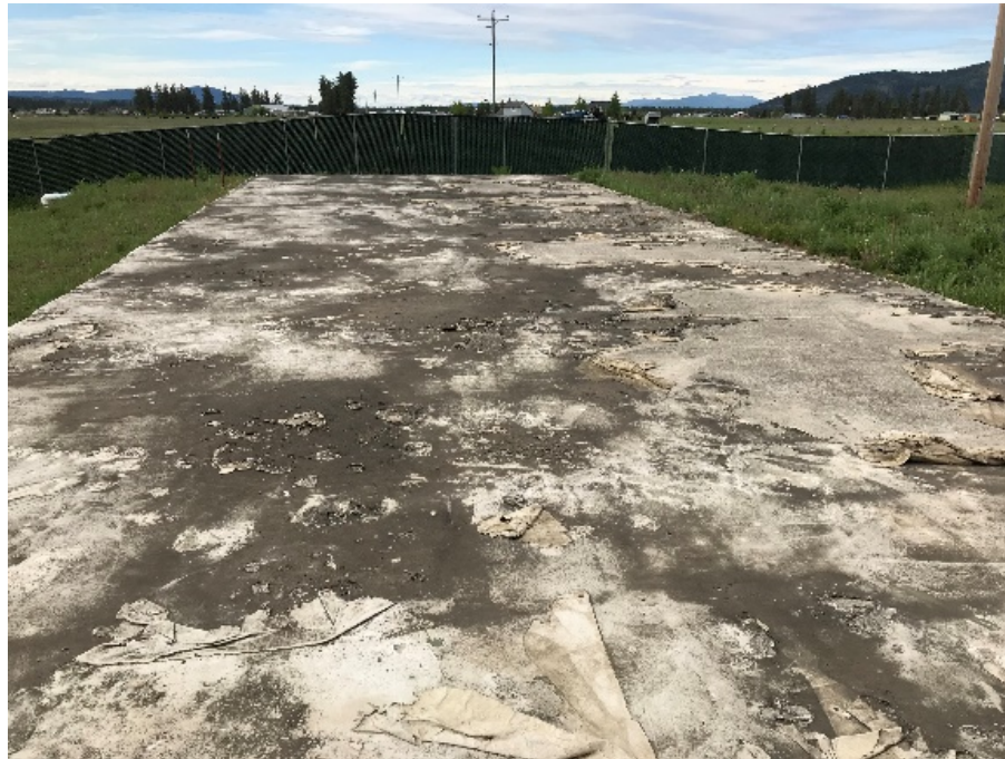
Top of Reservoir
