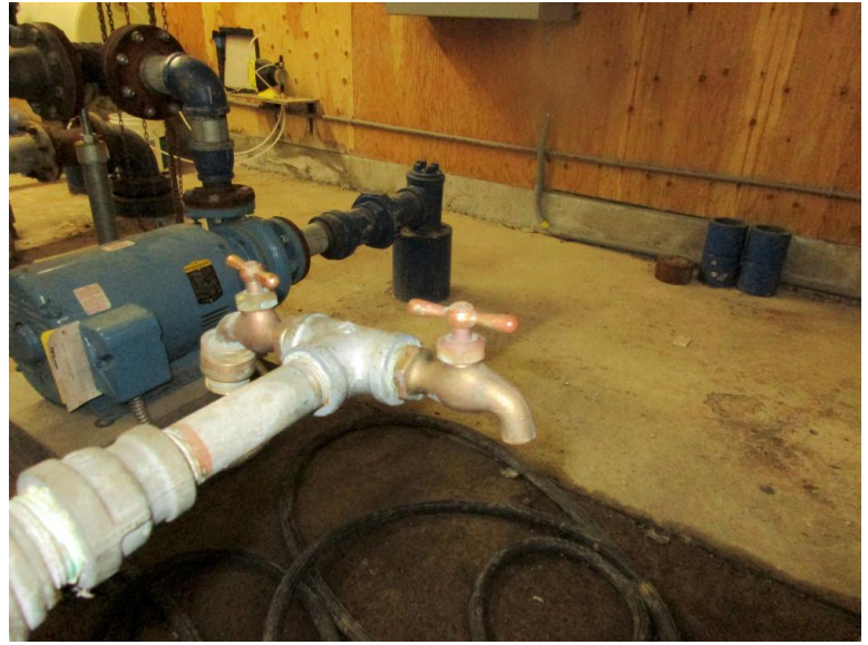
Photograph 12: Smooth nosed sample tap
