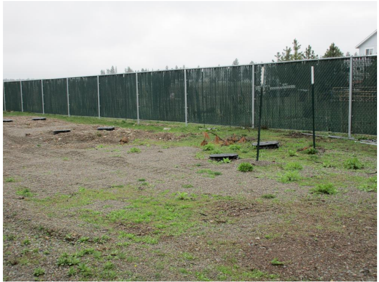
Photograph 2: Six underground propane tanks - 1000 gallons each
