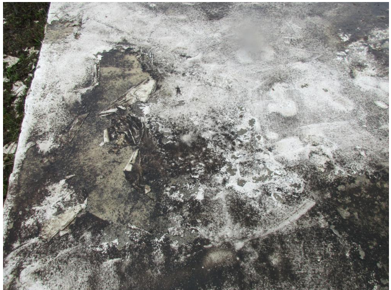
Photograph 4: Storage tank roof
